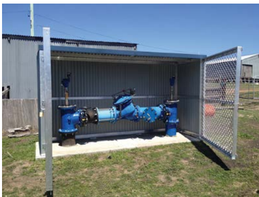
Above-ground Pressure Reducing Station Planning
