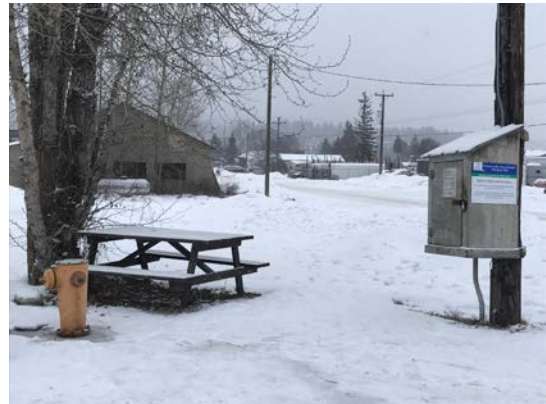
13 th Street Well Investigation
