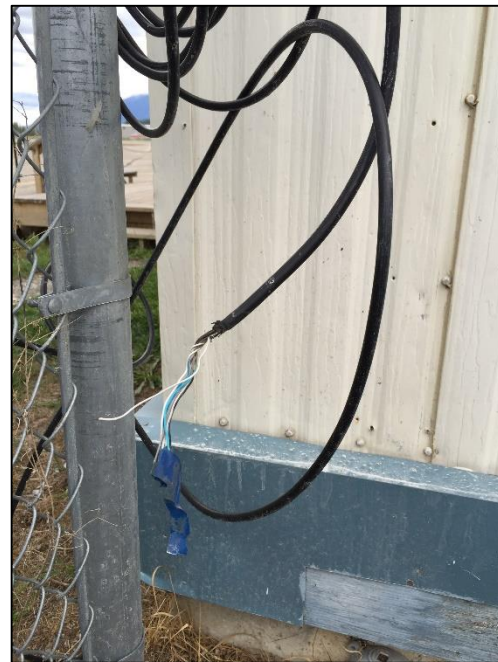
Photo E7 - exposed wire
