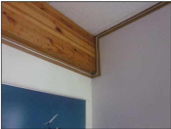
Photo A41 - laminated wood beam
