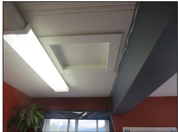
Photo B24 - ceiling access hatch
