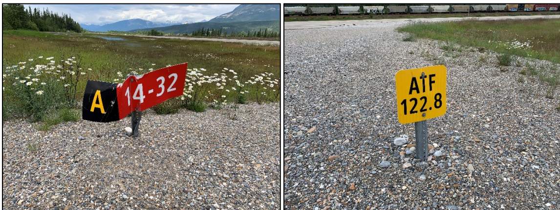
Damaged (left) and undersized (right) airside signage
