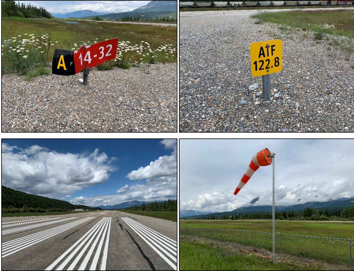
Airfield signage (top), pavement markings (bottom left), and a WDI (bottom right)
