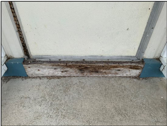
Crawlspace vent improperly covered
