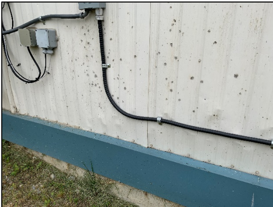
Buckling and surface condition of metal cladding
