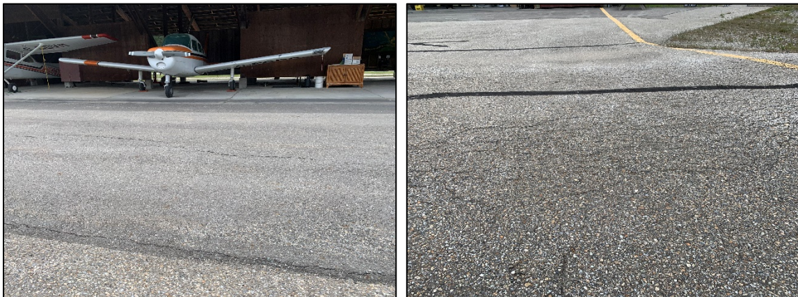
Apron I: Low severity unsealed cracks (left) and weathering (right)
