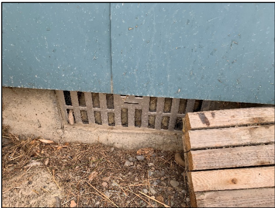
Crawlspace vent improperly covered
