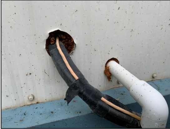
Partially unsealed openings in building wall
