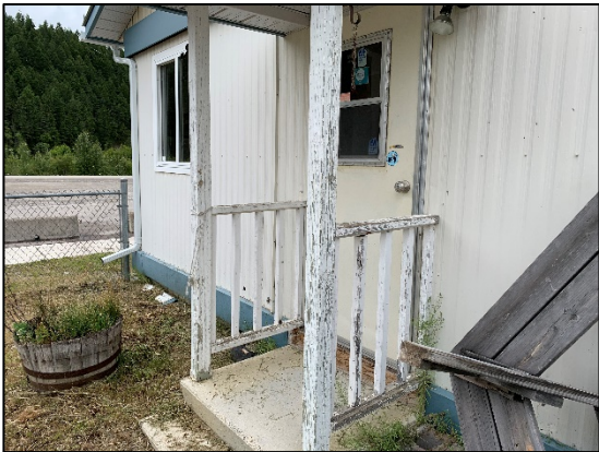
Weathered entryway railing and roof supports
