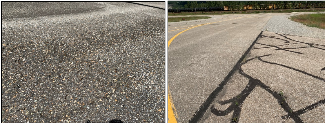
Taxiway B: Pavement weathering (left) and sealed cracks along the interface with Apron II (right)
