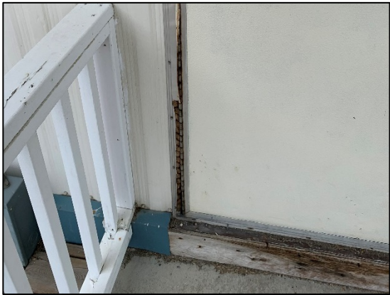
Door hinge is rusting and exposed
