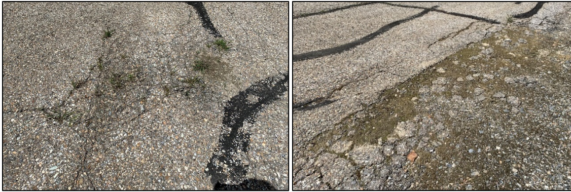
Apron III: Vegetation growth (left) and high severity alligator cracking (right)
