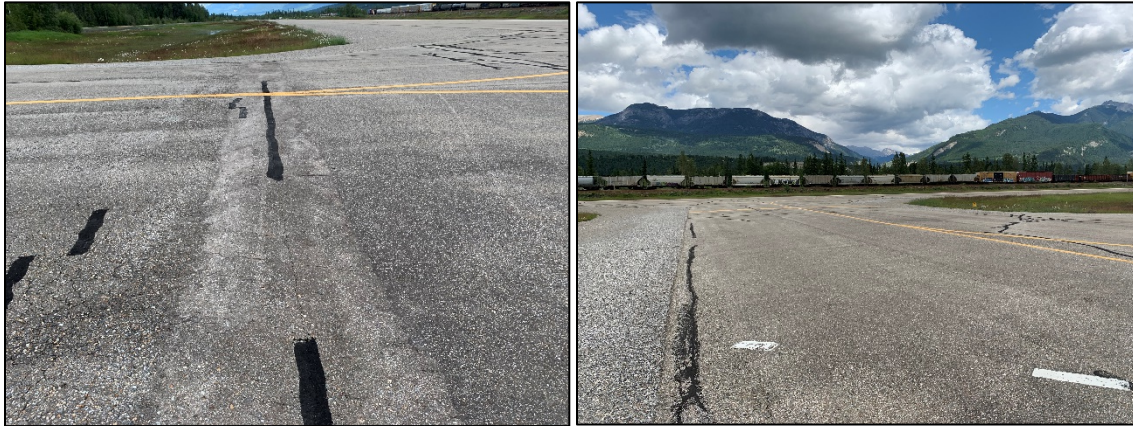
Taxiway A: Partially sealed transverse crack (left) and longitudinal cracking (right)
