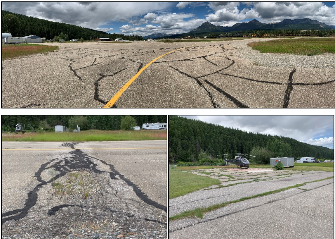
Apron II: Surface distresses (top), culvert pavement breakup (bottom, left) and vegetation growth (bottom, right)
