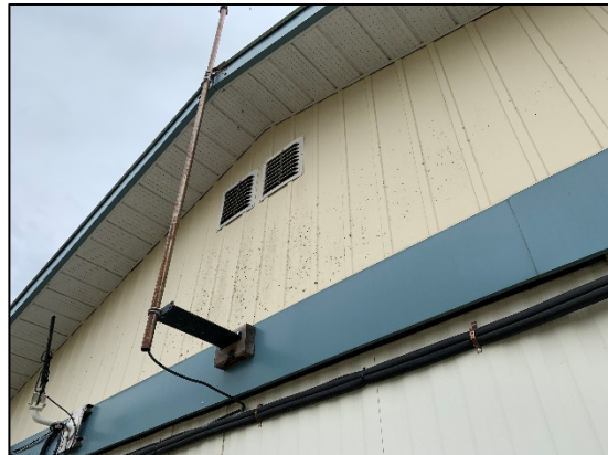
Buckling and surface condition of metal cladding
