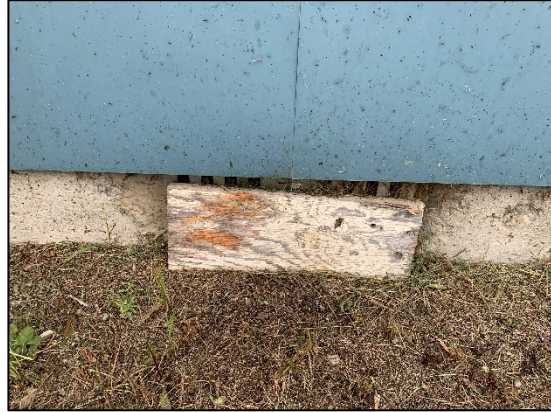
Crawlspace vent improperly covered
