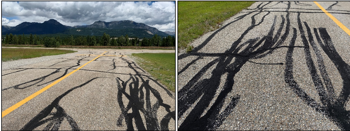
Taxiway C: Longitudinal cracking along the taxiway edges
