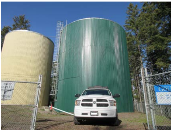
Reservoir ROV Inspections
