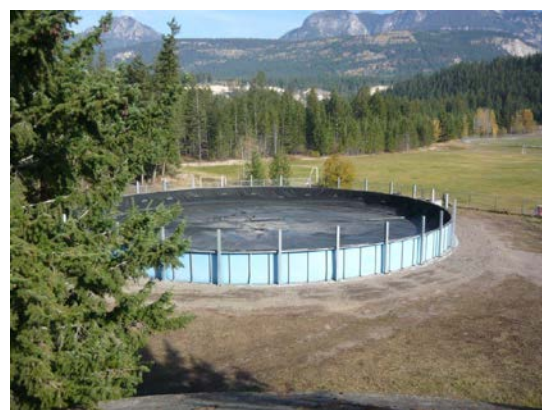
Hypalon Reservoir Liner Installation
