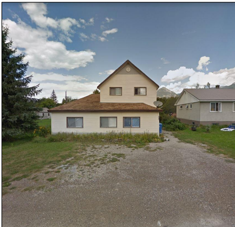
Existing House / Front Yard
