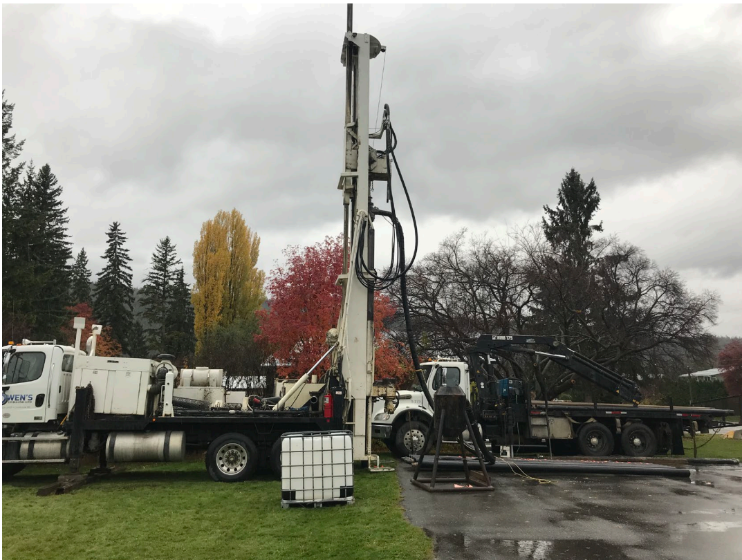
Well 7 Drilling Set-up
